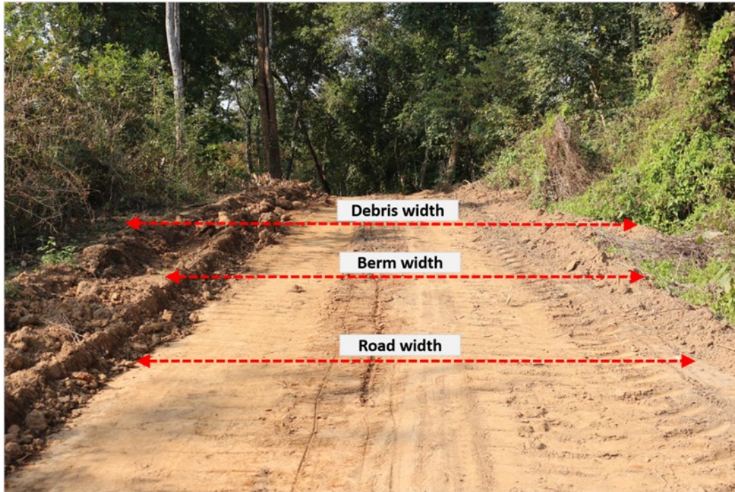
Figure 2-2 Measurements of the road width, berm width and debris width
