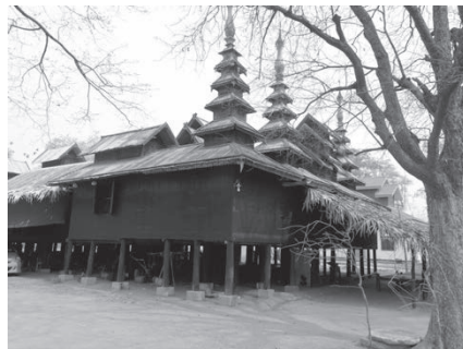
Fig.3.165. Taw-Way-Kan Kyaung Building 1 25
