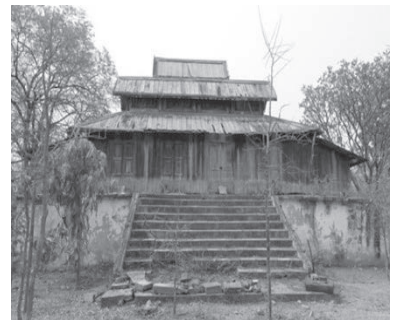
Fig.3.166. Taw-Way-Kan Kyaung Building 2 25
