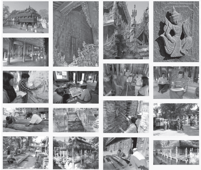
Fig.2.11. Shwe-Nan-Daw Monastery's Restoration Works *10
