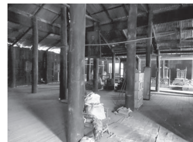
Fig.3.175. Vulnerable Conditions in 2 nd Floor of Khan-Taw-Taung Kyaung* 5
