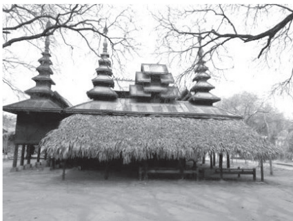
Fig.3.164. Taw-Way-Kan Kyaung Building 1 25
