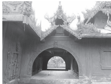
Fig.3.81. Arched Connecting Passage-way of Shwe-In-Bin Kyaung *4
