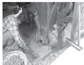
Fig.2.8. Repairing of Dragon-Serpent (Nayar) sculptures *3
