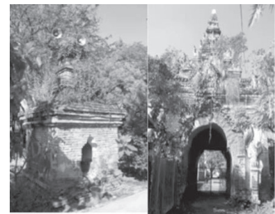
Fig.3.104. Existing Brick Gate of Medaw Kyaung: Queen Mother’s Monastery *5
