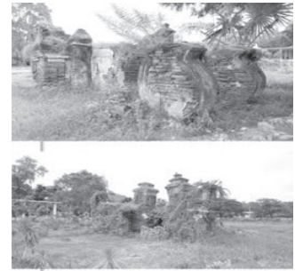
Fig.3.64. Remains of Brick Stairs* 5
