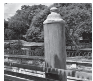
Fig.2.9. Replacement of New Teak Wood Pillar *5
