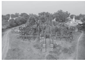
Fig.3.159. Existing Conditions of Pakhanng Kyaung 25
