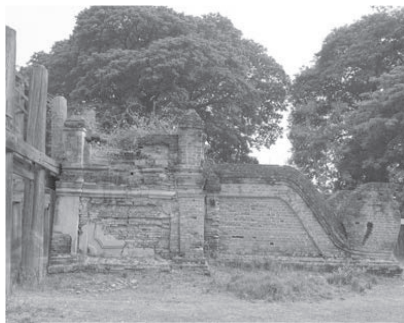
Fig.3.162. Existing Brick Stairs of Pakhanng Kyaung 25
