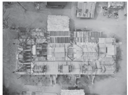
Fig.3.163. Top view of Taw-Way-Kan Kyaung Building 1 25
