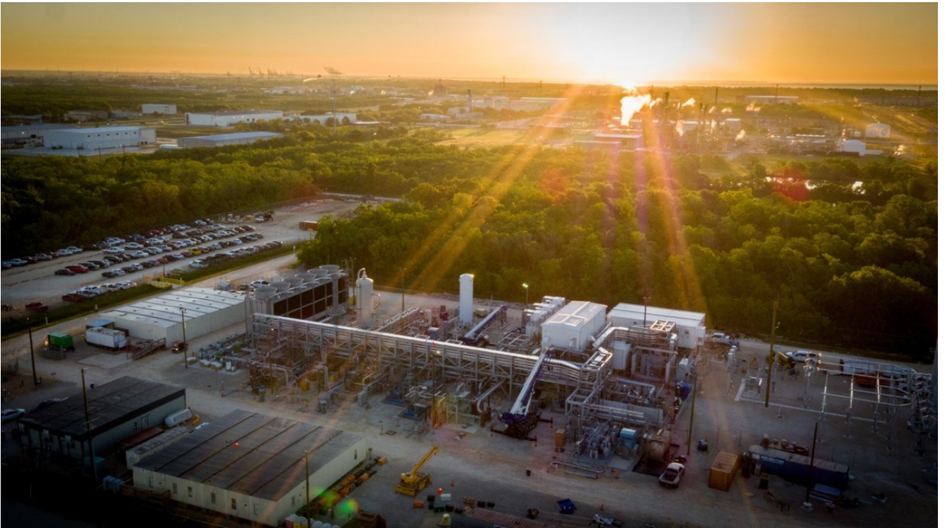
Fig. 6: NET Power's supercritical carbon dioxide power cycle demonstration plant (Courtesy of NET Power and McDermott)[18]
