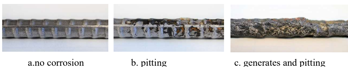
Fig. 5.12—View of surface corroded steel bar after removing corrosion products
