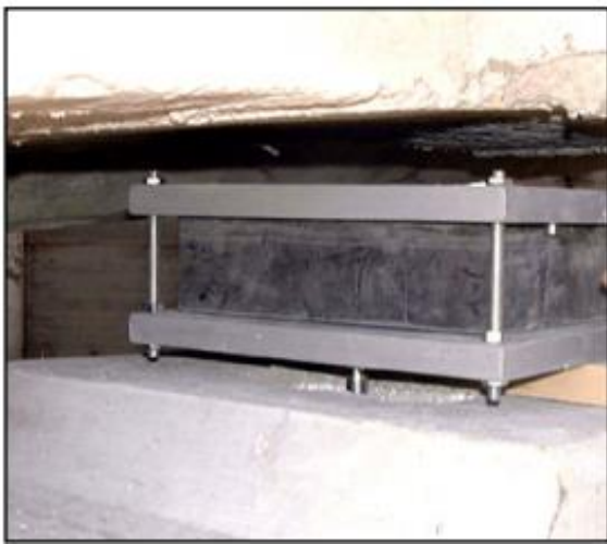
a. Elastomeric bearing with anchor plate
