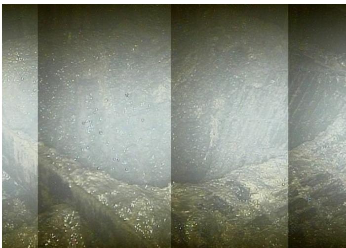
Figure 5.3 Meter-wide Hole in Grate Below Pressure Vessel in Reactor 2, Possibly Caused by Melted Nuclear Fuel (As of 6 February 2017)
