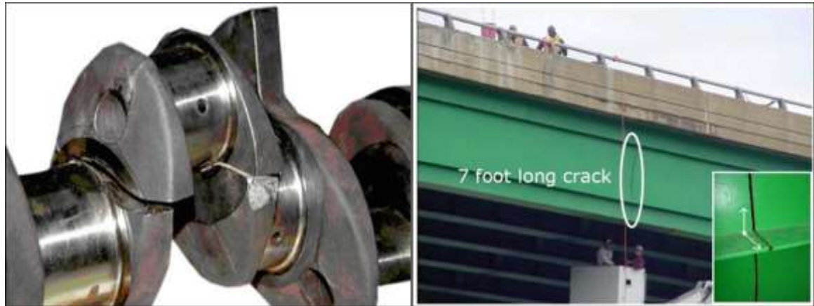
Fig.1.1 (a) Fatigue failure of engine crankshaft [2], (b) Fatigue cracking on the bridge girder [3]
