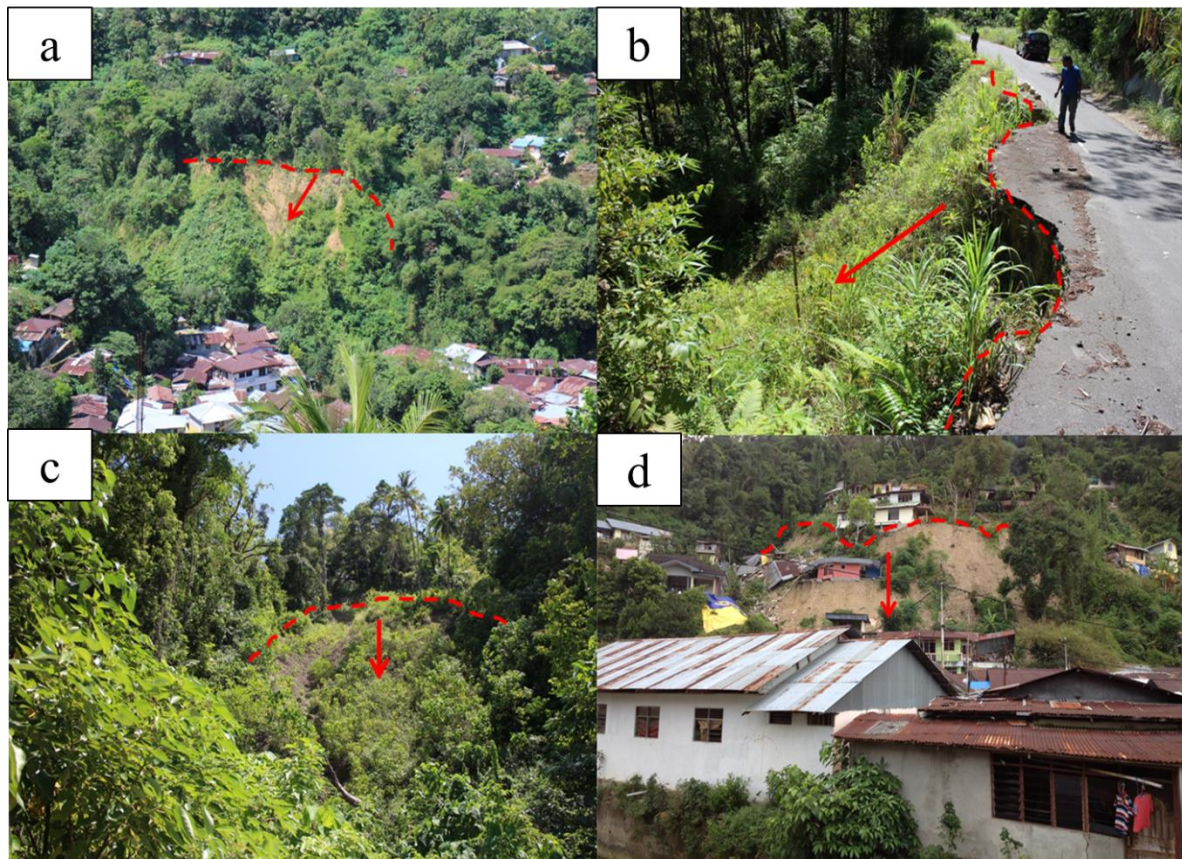
Figure 3.1 a) landslides near settlement area; b) landslide along the road network; c) landslide case in the Ambon volcanic rocks geology, d) houses affected by landslides.
