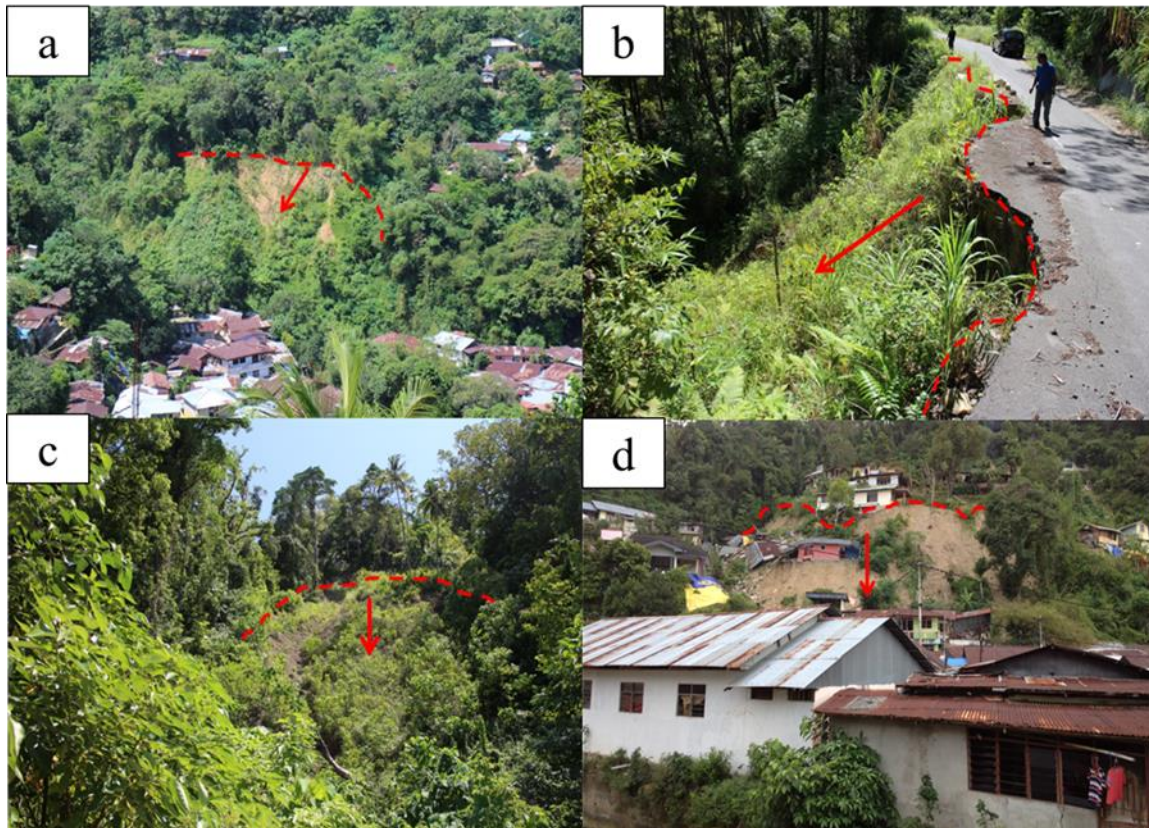
Figure 4.1 Landslide cases found during field investigation in 2015 a) landslides near settlement area; b) landslide along the road network; c) landslide case in the Ambon volcanic rocks geology, d) houses affected by landslides..
