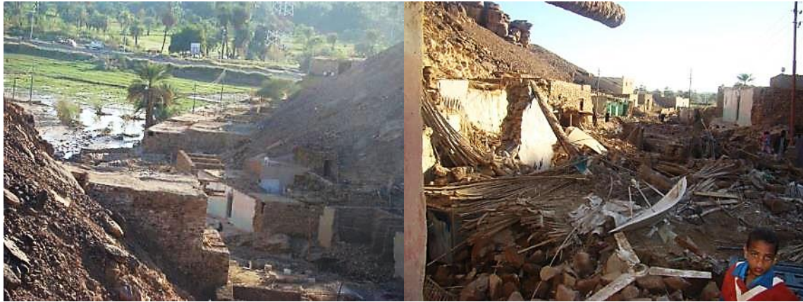
Figure 3-3 Buildings were destroyed in Abouelreesh village after a torrent in 2010.
