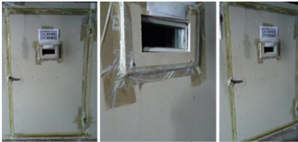
Figure 4-15 Water condensation observed on the window
