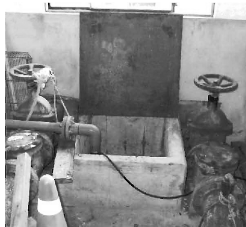
B : The entrance of the water storage tank.
