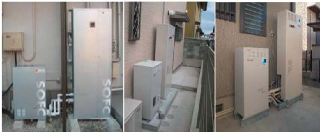
Figure. 1-7. Appearances of installation sites of residential SOFC combined heat and power systems under demonstrative research project in Japan [16].
