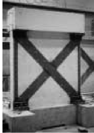
Figure 3.4 Vertical and diagonal steel bracing [11]
