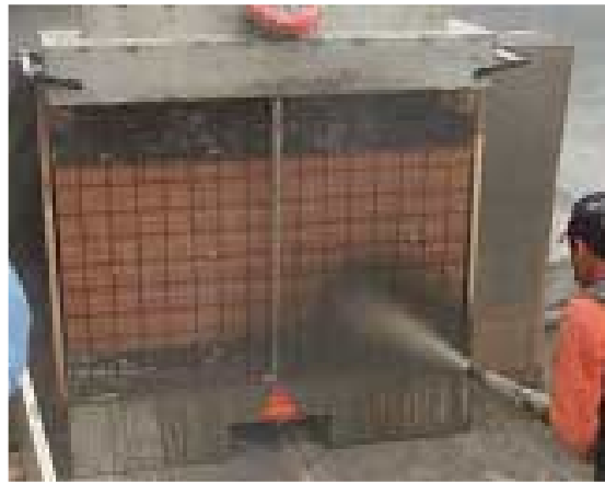
Figure 3.2 Externally retrofitted wall in shotcrete method [11]
